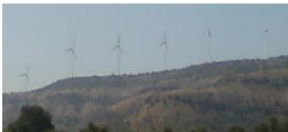
Fig.14- Wind Farms near Dewas Ujjain, India
